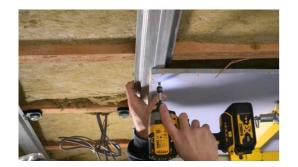
8. While holding the acoustic plasterboard in position, use the 25mm self-drilling screws to secure the board into each ReductoClip furring channel. Screw the fixing in place until the screw head is flush with the plasterboard. A screw should be used every 200mm on each furring channel. Once the first plasterboard is in position, apply the next board butting up tightly to the previous board and continue.
